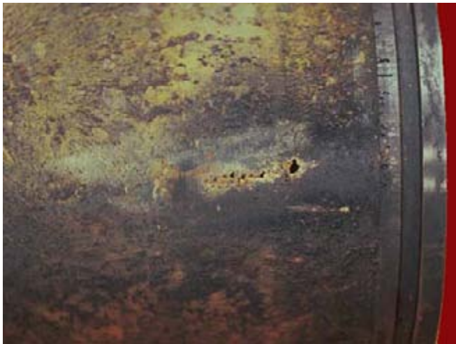
Fig. 40: Cylinder liner walls with heavy external scale may have areas that are free of scale and are experiencing cavitation-erosion induced pitting corrosion.
